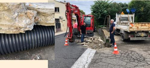
Work to bring the road into compliance carried out at the Pressoir was roundabout on the Chemin de la Montagne. The rainwater drainage system has been restored and the retention basin is finally operational again.
